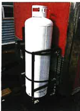
#4 Propane tanks MUST be secured
